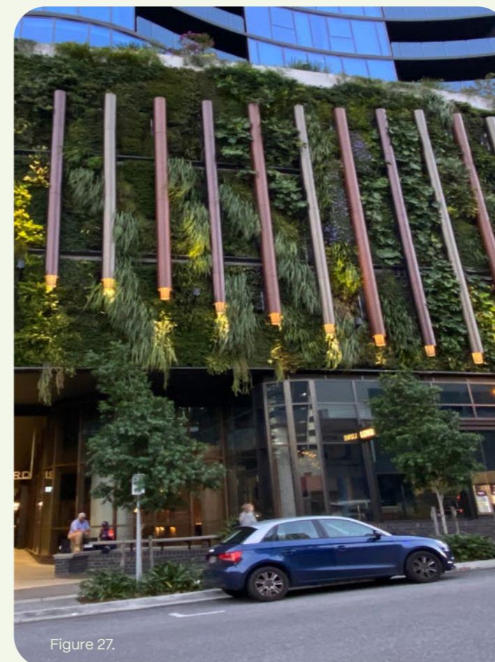
Figure 27. Integrated green walls at the streetscape level offer internal cooling and within the public domain. West End, Brisbane, Queensland. Figure 28. Green walls can be used to hide unattractive blank spaces. Royal Adelaide Hospital, South Australia.
