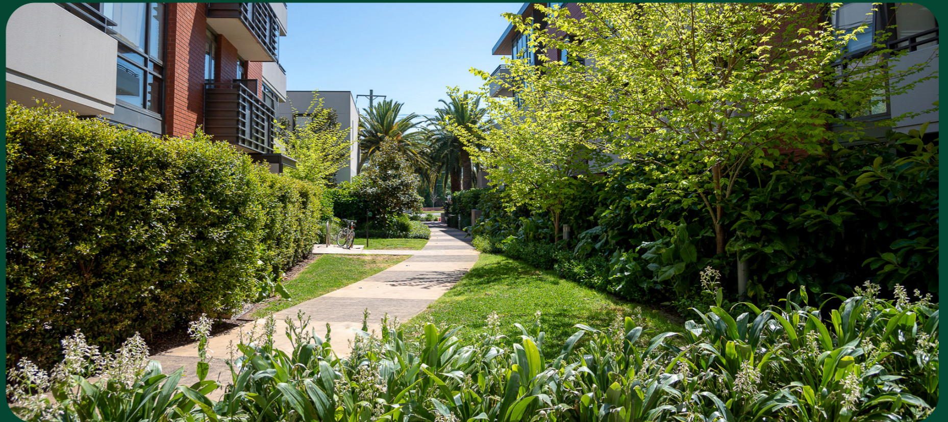
Figure 23. The ground level gardens at Caulfield Heath are constructed over a basement car park, Victoria.
