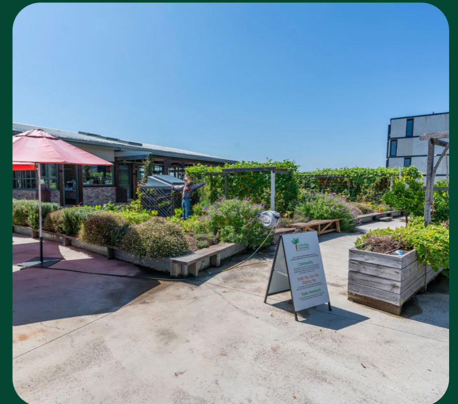
Figure 35. Productive gardens on the roof of the Burwood Brickworks Shopping Centre
