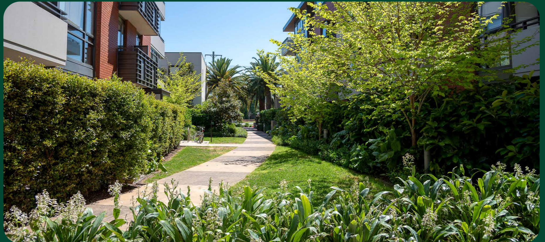
Figure 23. The ground level gardens at Caulfield Heath are constructed over a basement car park, Victoria.
