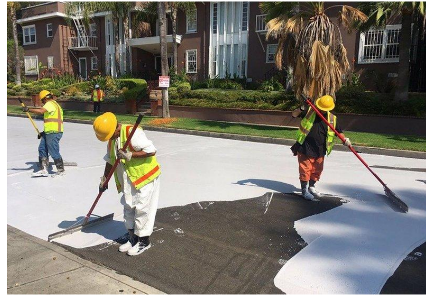
Figure 13: Cool pavement project in Los Angeles (14)
