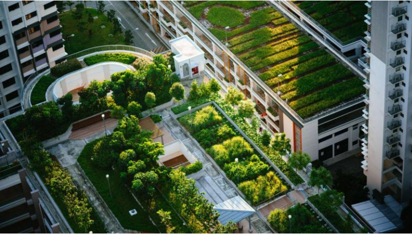
Figure 8: Example of green roofs (11)
